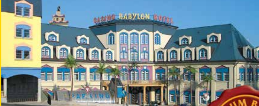
ALL UNDER ONE ROOF
