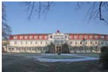
Spa pavilion in Bohdaneč
